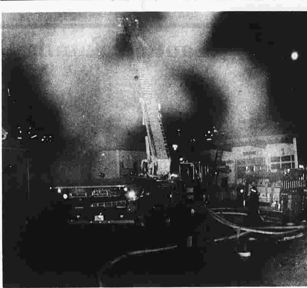
General alarm fire at E.F. Houghton and Co., 44 Stock Place, Manchester, early this morning heavily damaged the office and storage buildings at the facility. Firefighters and equipment from Manchester, Bolton, Vernon and South Windsor responded to the alarm. (Herald photo by Burbank)
